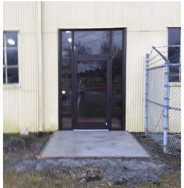
The Museum's public access door installation is complete!
