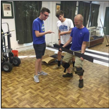
Museum members John William and Andrew Davis put the finishing touches on the floor of the community room/Ready Room for Andrew’s Eagle Scout project.
